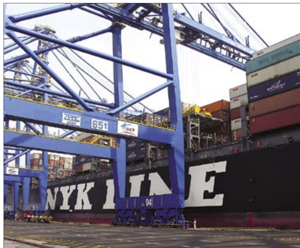
NYK's International Container Terminal at Dalian.
